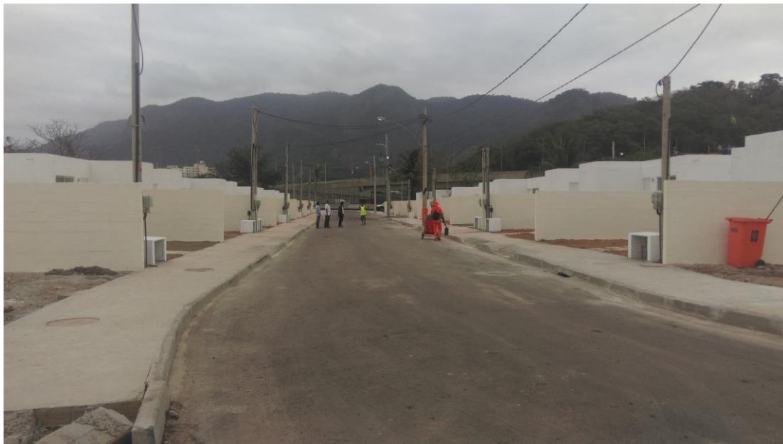
Figure 6.1: The new homes of Vila Autódromo. July 2016.
