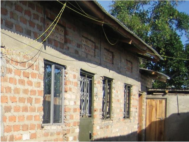
Figure 2. Permanent ventilators on windows and doors
