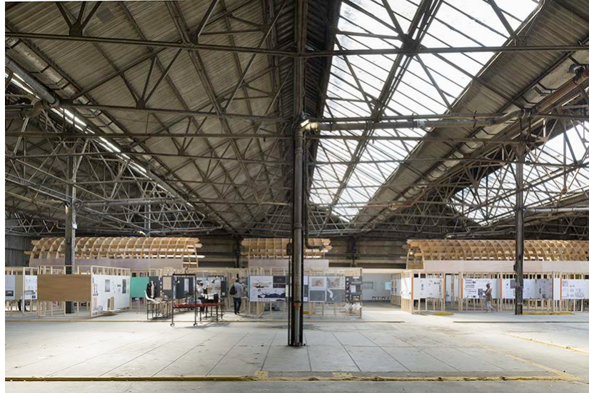
Figure 8. Reciprocating Lamella Roof pavilion rebuilt in 2014. Image courtesy of Jim Stevenson.
