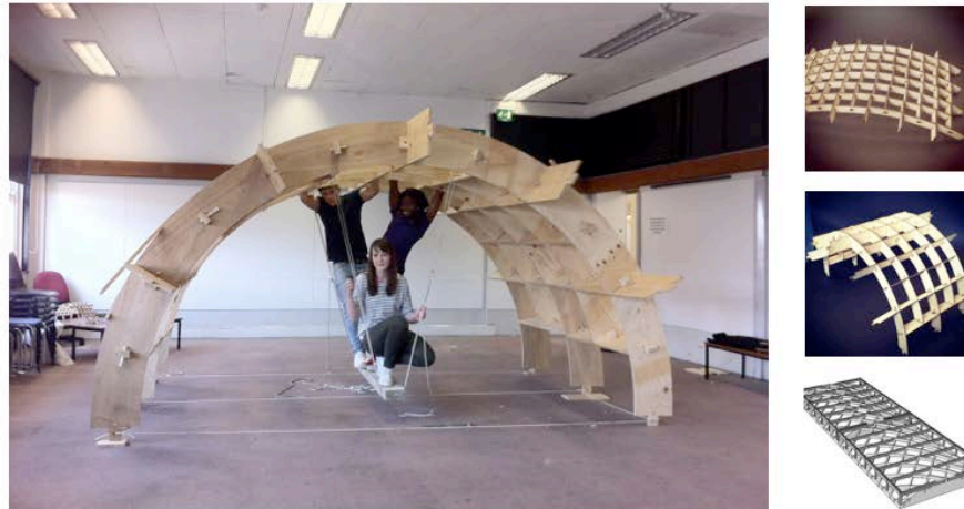
Figure 6. Reciprocating Lamella Roof. 17 Images Courtesy of Glenn Longden-Thurgood.
