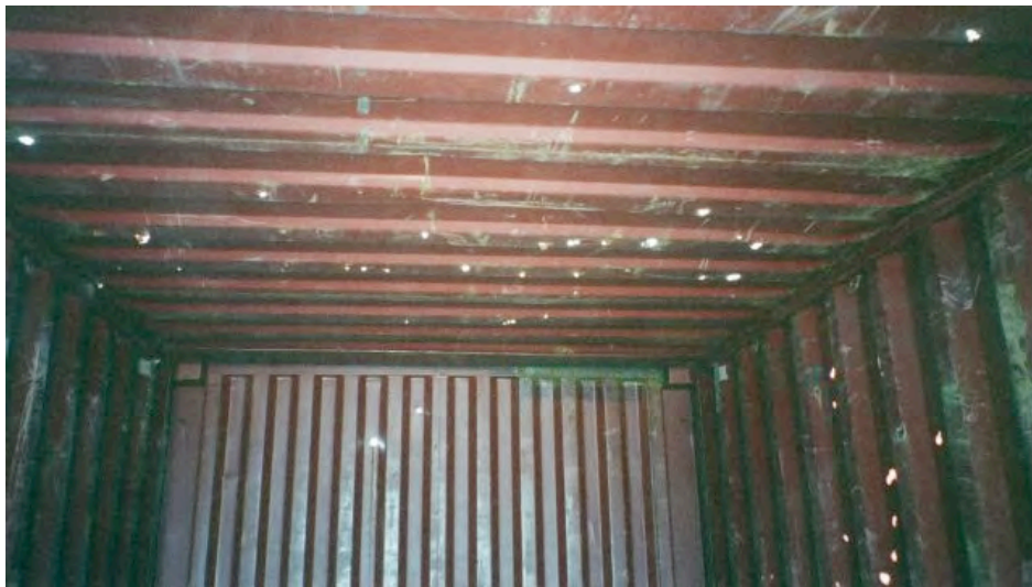
Case study1. The Flight (2003). The container prior to the installation
