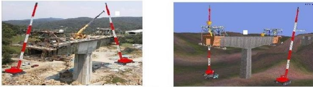
Figure 1: Difference between AR (left) and VR (right) for a construction project (Behzadan and Kamat, 2005)
