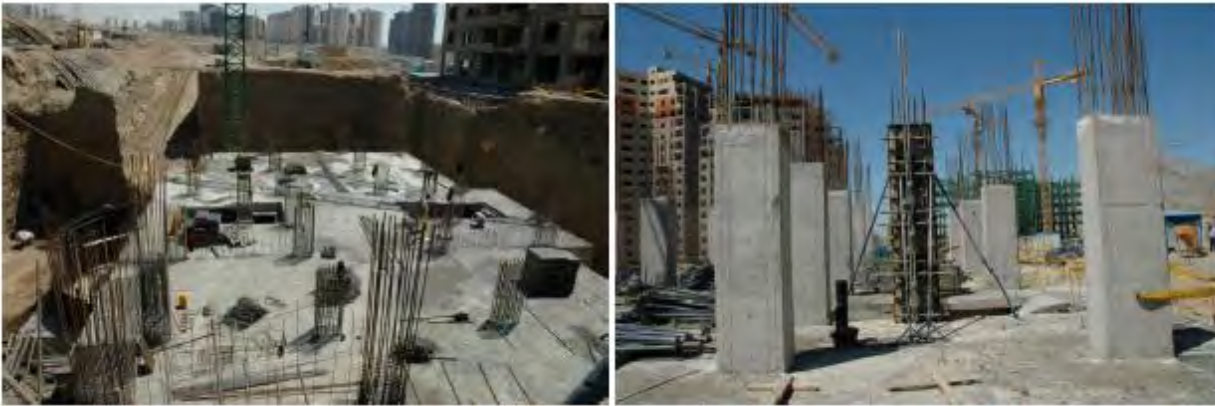
Figure 1: Construction methods in Iran.
