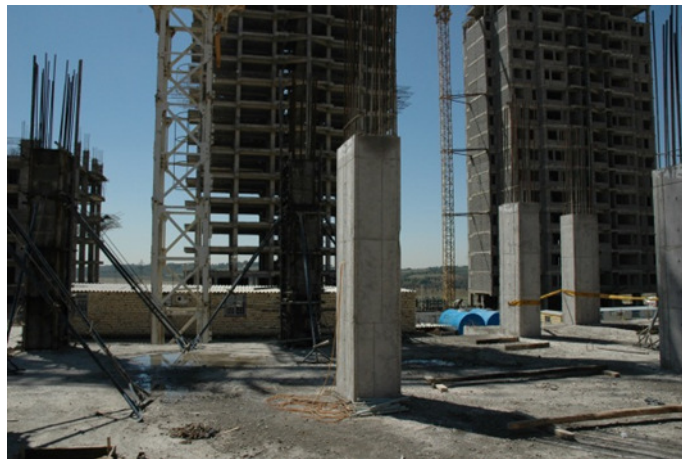
Figure 5: Construction methods in Tehran (RC frame); Source: the authors
