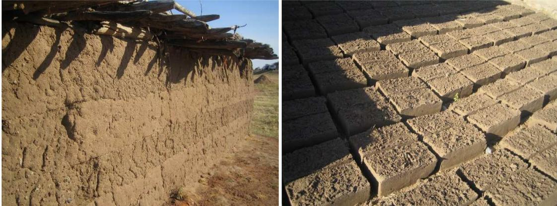
Figure 7. Cob construction (left) and adobe (right) construction. Source: The authors.
