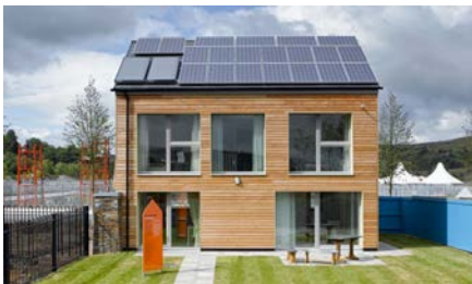
Figure 8 The 'Larch' Passivhaus Ebbw Vale (Jefferson Smith)
