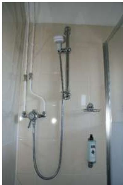
Figure 3: Typical shower cubicle in the upper floor guest rooms
