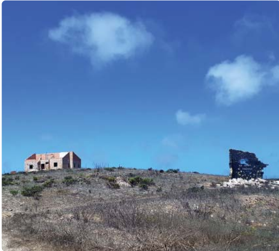
Ruin under renovation near Vila do Bispo
