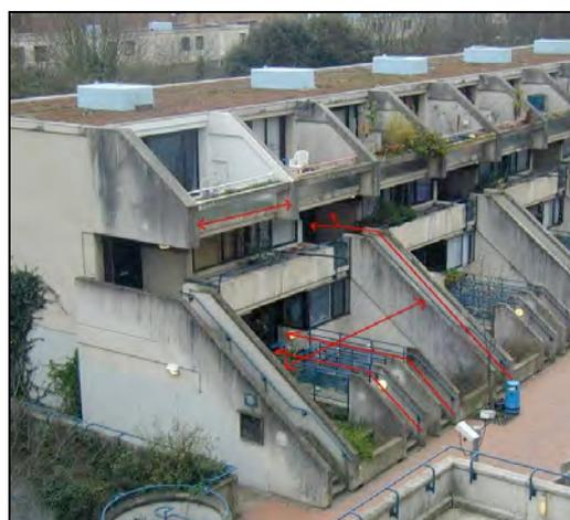
**Fig. 1:** View of block B, Alexandra Road. Red arrows indicate individual and shared entries to lower and upper maisonettes. The wider space below demarcates the shared 'forecourt' space of two units while the expressed cross-walls of the upper units identify individual units. One can also enter the lower level of the bottom unit in the gap between the parallel stair-bridges.
