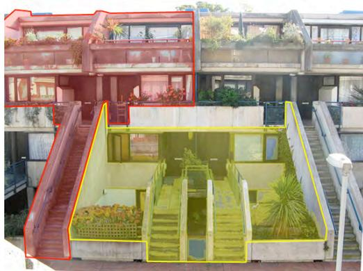
Fig. 24: Interlocking of paired units
