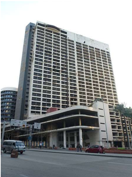
FIG. 24 The Holiday Inn, a still standing spectre of the conflicts in a sugar-coated area (source: Wikimedia Commons)
