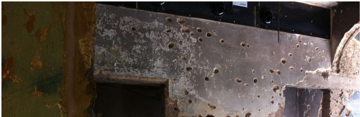
FIG. 13 An example of the smoothed, 'recreated' bullet holes on one of the walls inside Beit Beirut (source: HMA)
