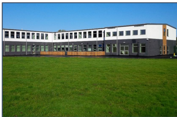
Figure 2.2: Example of prefabricated relocatable module and rooftop airspace extension designs. The relocatable module are used as an education facility, whilst designed as a permanent structure, any requirement to move or deconstruct the structure can be done so with minimal effort and cost
